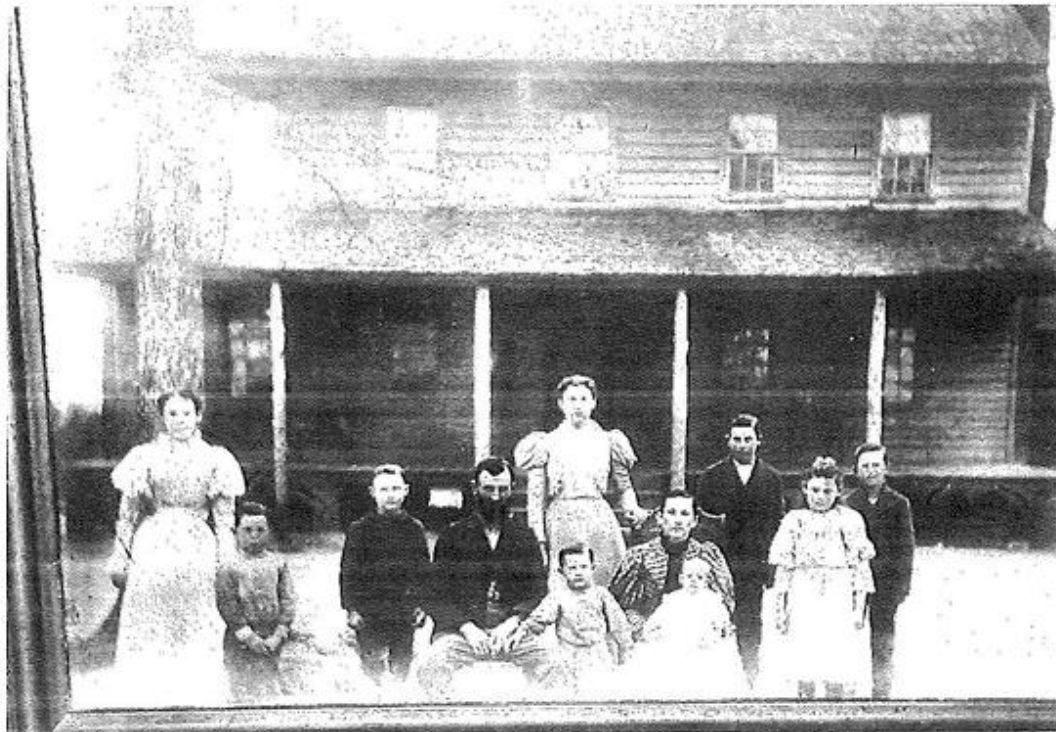
Photograph of the Yarborough House provided by F. G. Scurry.
