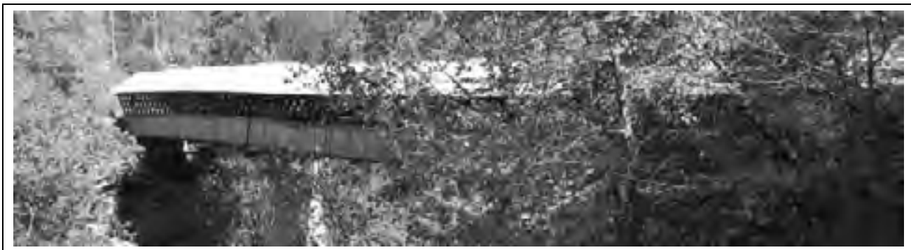
Swann Covered Bridge, Cleveland, AL (photograph by Leonard Yarborough)
