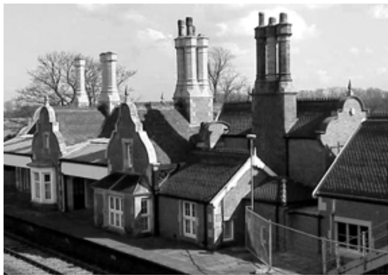
The Bocklesby railroad station, built for the Earl of Yarborough's estate
