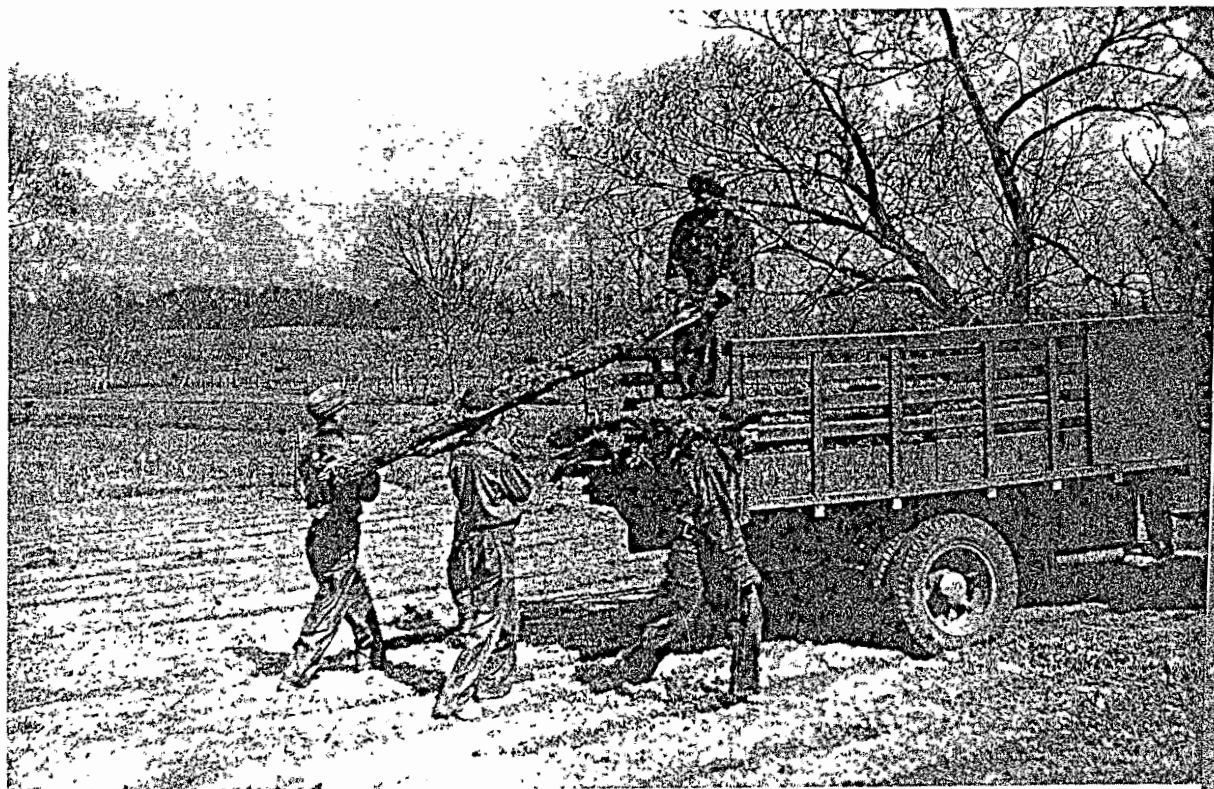
OPHELIA KESSEER YARBROUGH HISTORIAN BOX 261 NEWCASTLE, TX 76372 ...lees loading Bermuda sod on boards for hauling to terrace outlet channels.
